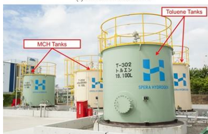
(b) Tank yard
